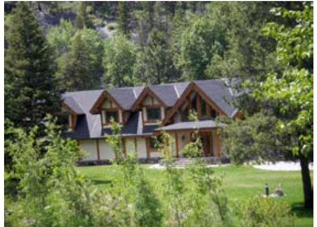
This home has non-flammable roof, rock foundation, irrigated lawn, and there is a river directly behind the home to serve as a water source in an emergency.
