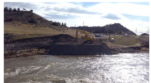
Drill Rig Equipment Pad (east side)
