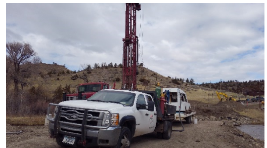
Drill Rig Subcontractor On-site
