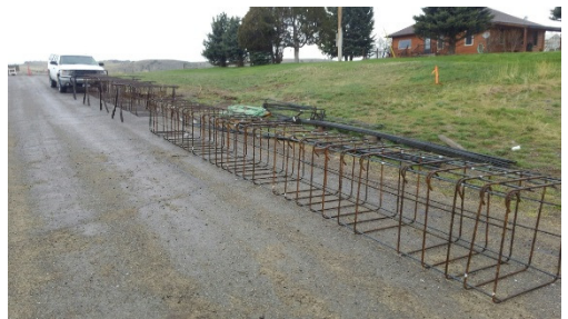
Abutment Rebar Cage
