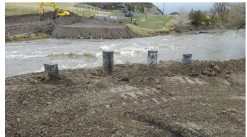
Drilled Pile Casings at West Abutment
