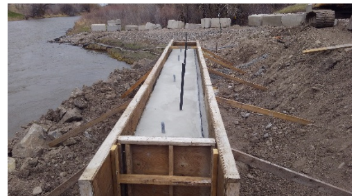
Curing concrete cap on the east abutment
