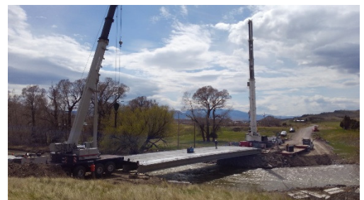
Concrete bridge beams in place
