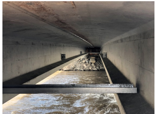
Steel bridge diaphragms to be installed
