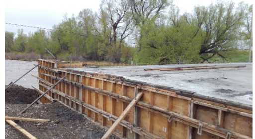
Curing concrete backwall and wingwall on the east abutment
