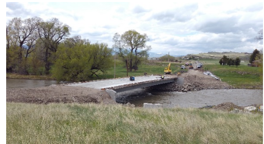
Bridge approaches built up
