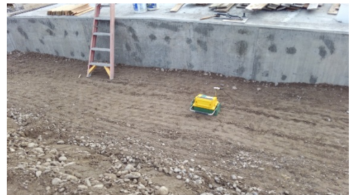
Backwall in place
