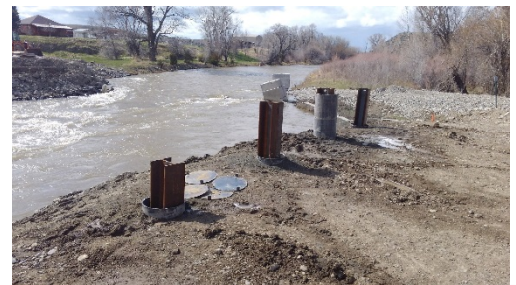
Driven piles encased in concrete
