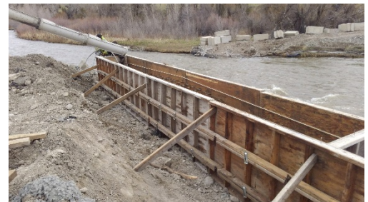
Pouring concrete for abutment cap
