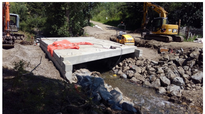
Placing Bridge Approach Material
