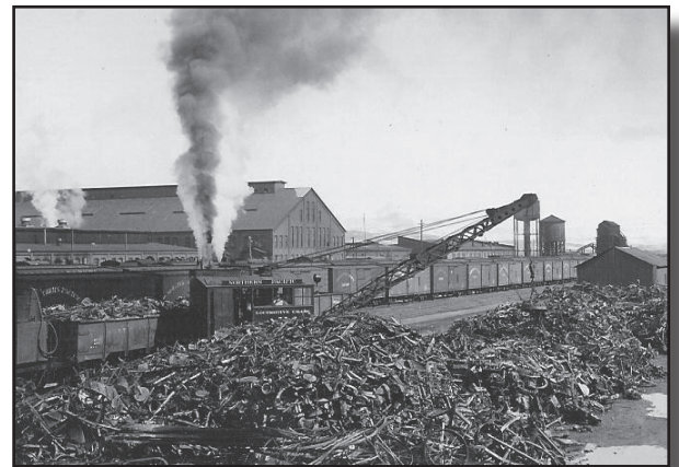
The crane and piles resulting from citizens' efforts during the 1943 WWII scrap metal drive.
