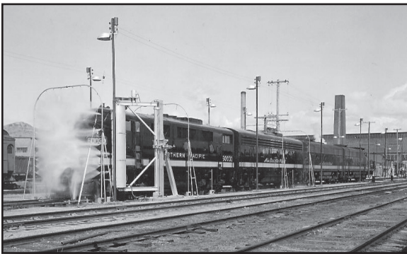
New Diesel Engine Washer, March 27, 1958.
