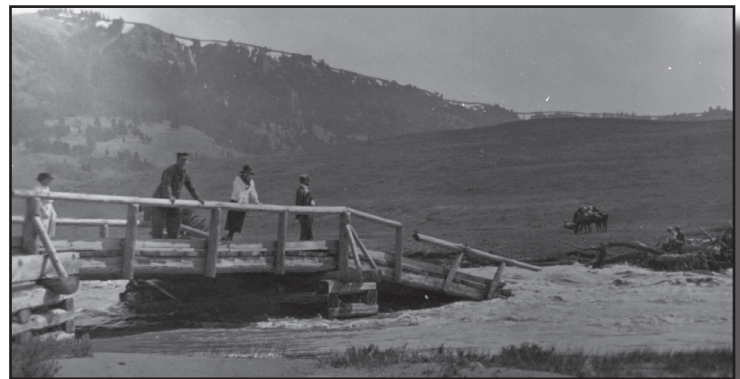
Visitors at the washed-out Lamar River Bridge in northeastern Yellowstone National Park
