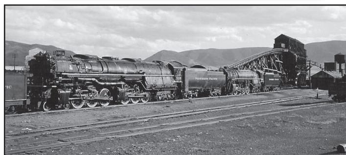
Top: Stationary or Power Plant, June 21, 1946. Bottom: Locomotive in front of the coal dock, June 1955.
