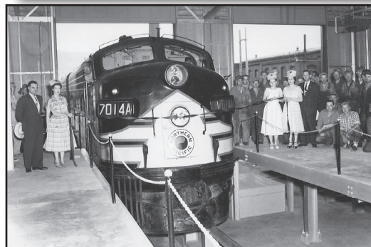
Above center photos: Dedication Day for the new Diesel Maintenance Shop, July 25, 1957.
