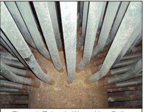
Figure 7. Tubes in Waste Heat Boiler
