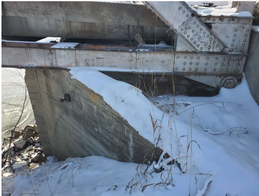
Figure 8: Truss resting on retaining wall.
