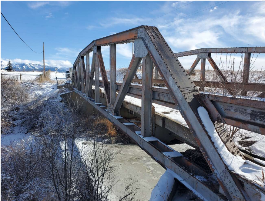
Figure 1: Horse Creek Road Bridge
