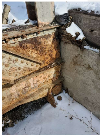
Figure 3: Movable bearing flush with abutment
