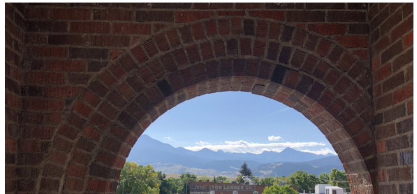
Brick arch on Elks Lodge balcony, Photo by MT CDC, 2023
