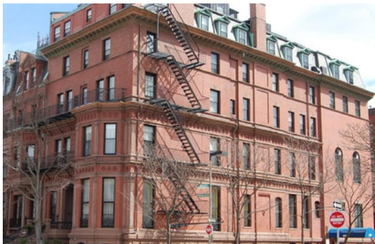
Chilton Club, New York, Ware and Van Brunt Architects
