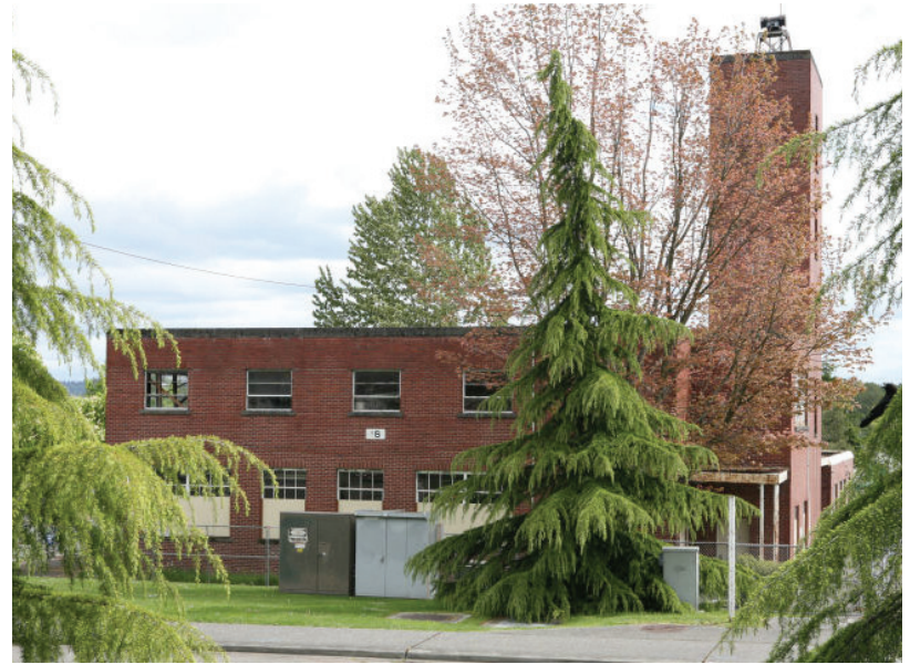
Julianna Ross, Building 18, view of west facade and hose drying tower
