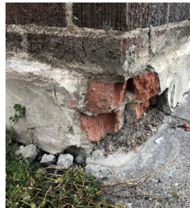
Bricks of the basement exterior wall as seen from the outside
