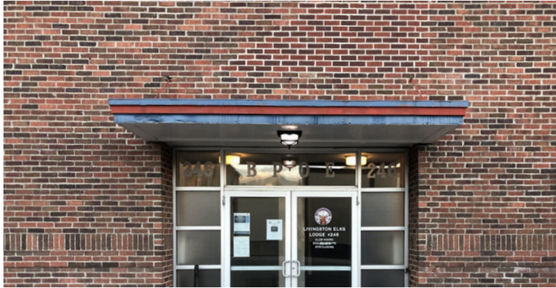
Area of brick replaced over the W Lewis St entrance
